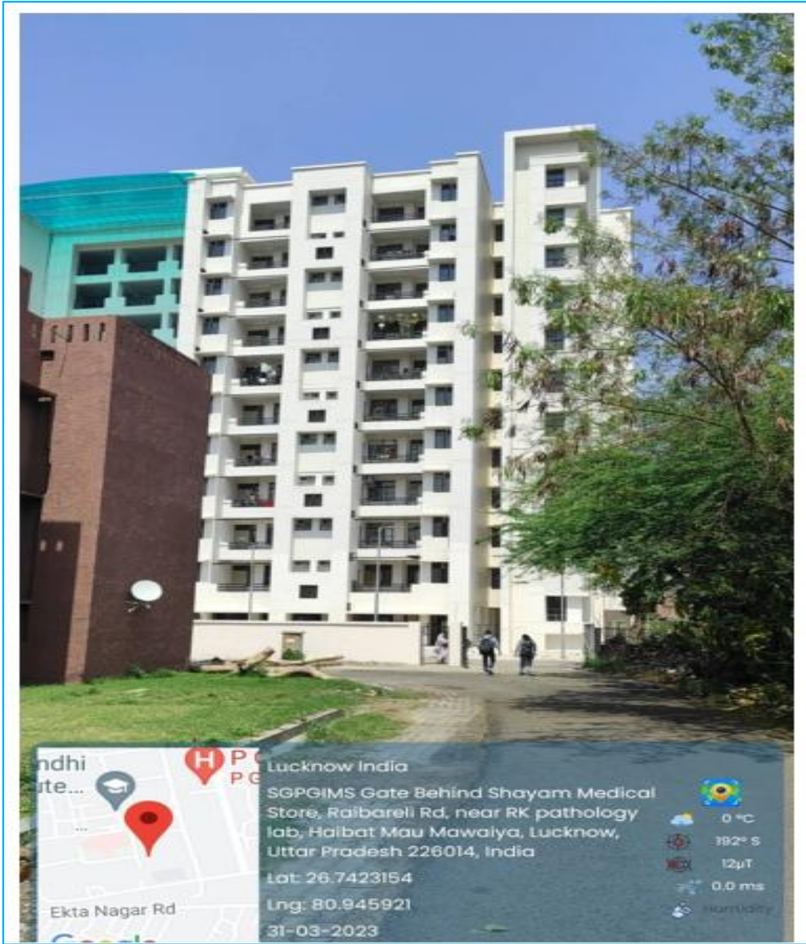
Multi-storeyed unmarried hostel for resident doctors
